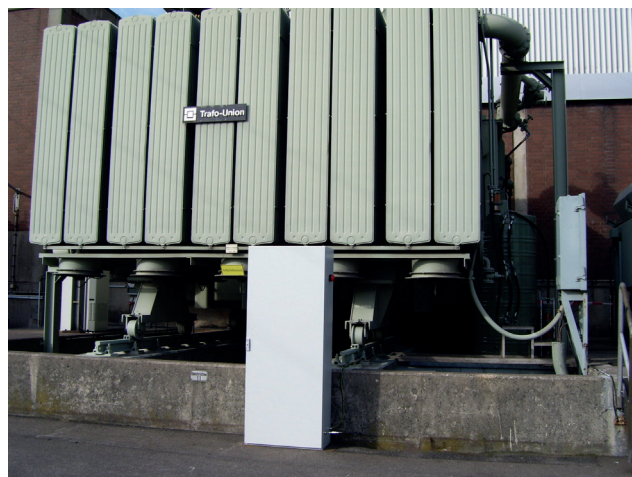
Figure 8: G3B unit with nitrogen supply
