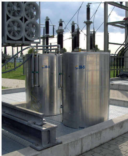
Figure 6: G3B unit with weatherproof lining
